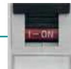
The green/red switch colour clearly indicates the connected/disconnected status.
